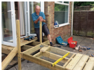
Building an access ramp.
